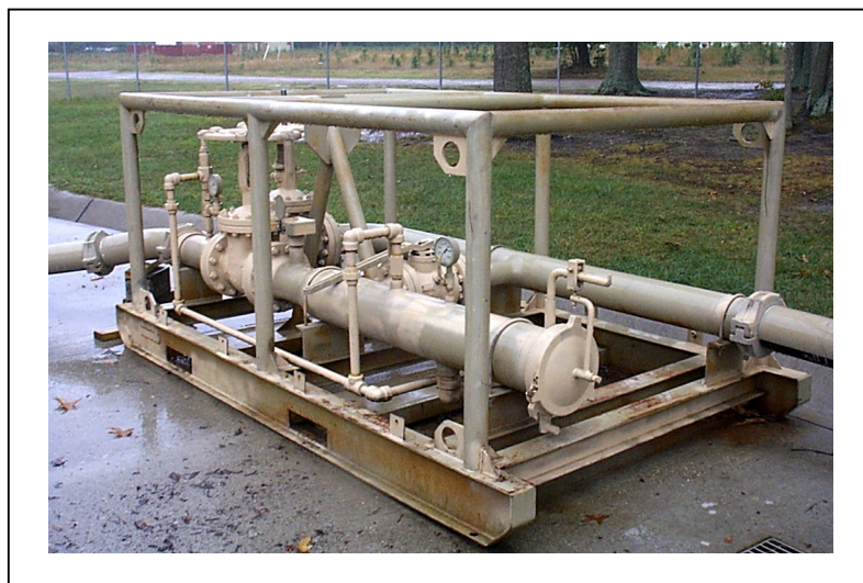
Figure 2-3. Launcher/Receiver assembly.
