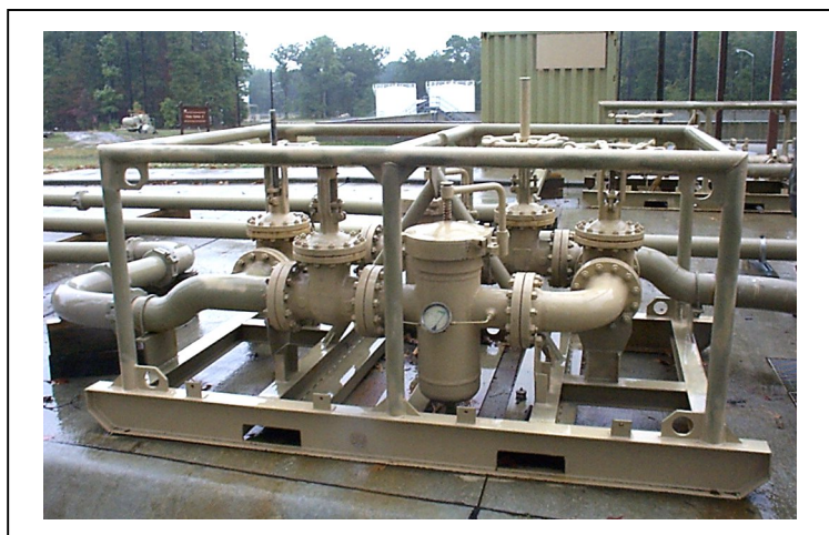
Figure 2-4. Strainer assembly.
