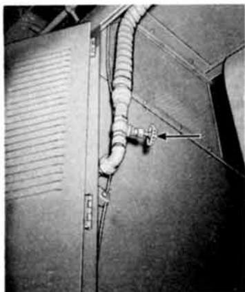
Fig. 27 Water Inlet Valve
